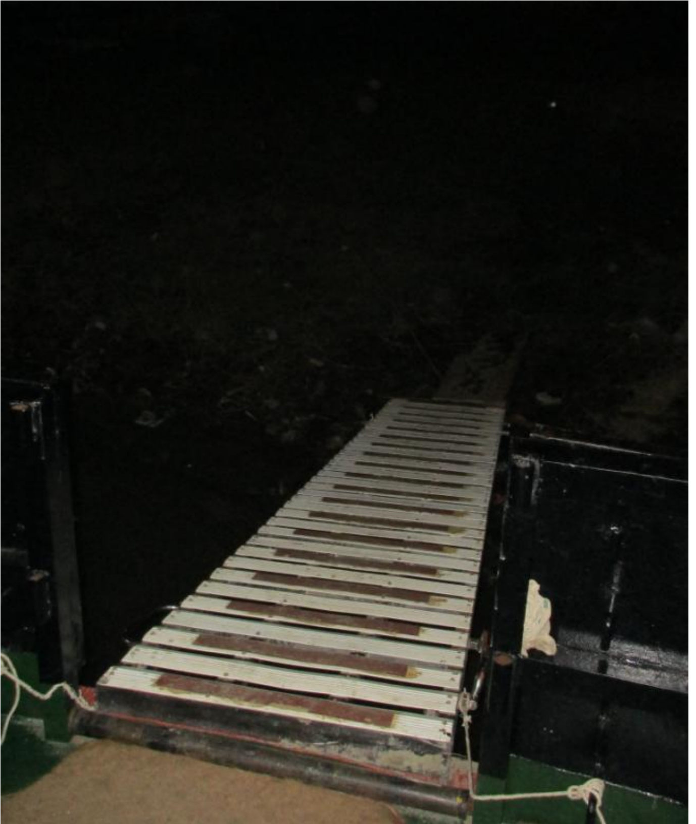
Example D: The gap between gangway and platform is a potential trip hazard.
