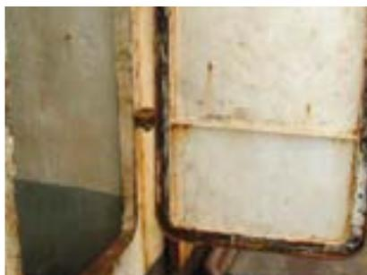
Figure 2: Poorly maintained access rubbers
